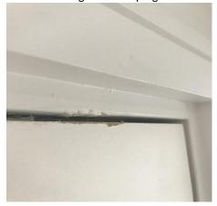
• Unpainted corner woodwork where lock latch recess has been chiselled into bathroom.
